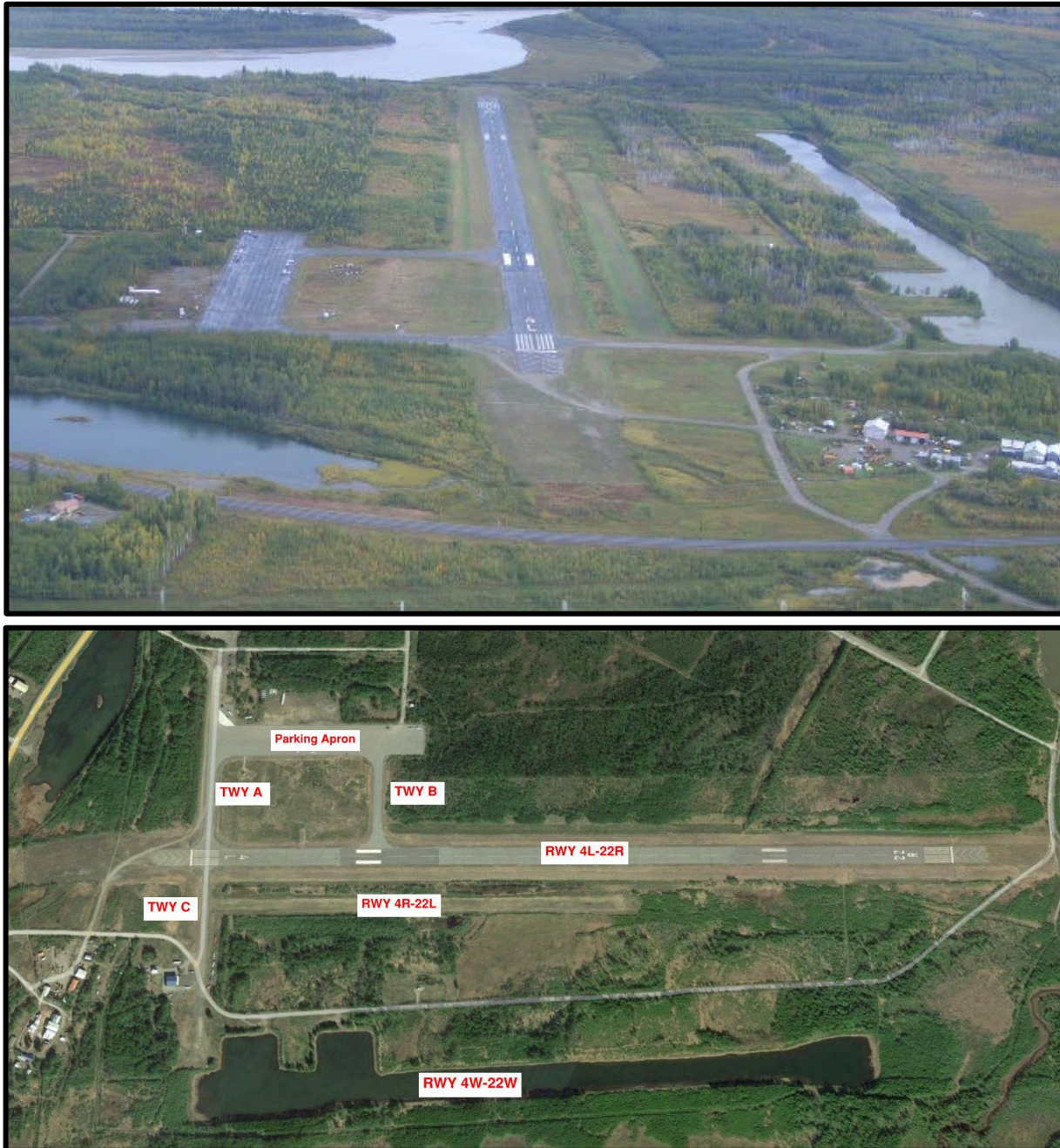
Figure 1.4: ENN Runways and Apron (Top: View from West, Bottom: Aerial)
