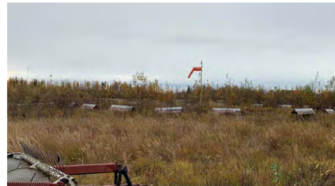
Segmented Circle and Windsock Deferred Maintenance and overgrown brush effect the performance and reliability or NAV AIDs
